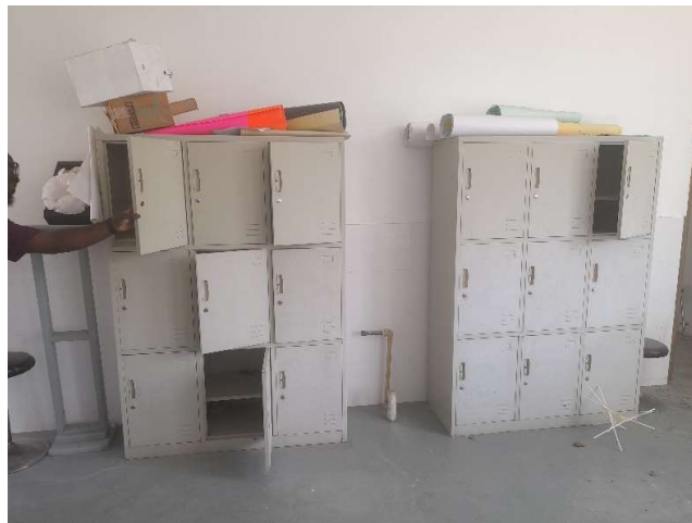
Picture 4. Lockers within classroom to be secured to wall
