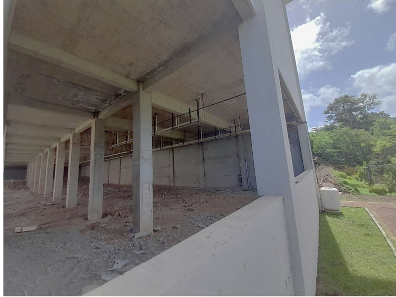
Picture 5. Cellar under classroom and lab with gas lines and plumbing
